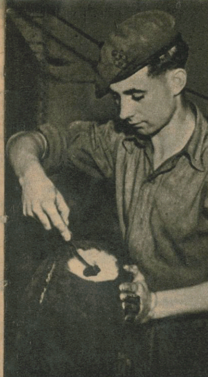
Craftsman B. E. Streeton prepares a tyre for vulcanising.
