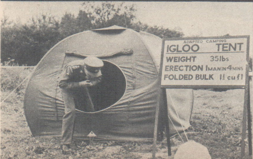
The experimental igloo tent is inflatable and held in position by rubber tubes. When deflated it fits into the kitbag beneath the sign board.
