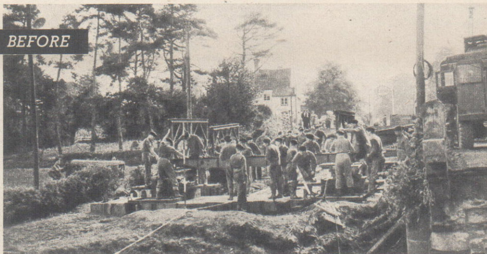
Above: Only a few hours after floods had swept away the bridge at Foston, Sappers from 30 Field Squadron, Royal Engineers were hard at work building a new one. Below: A 'bus was one of the first vehicles over the new bridge which is likely to remain in use for some years.
