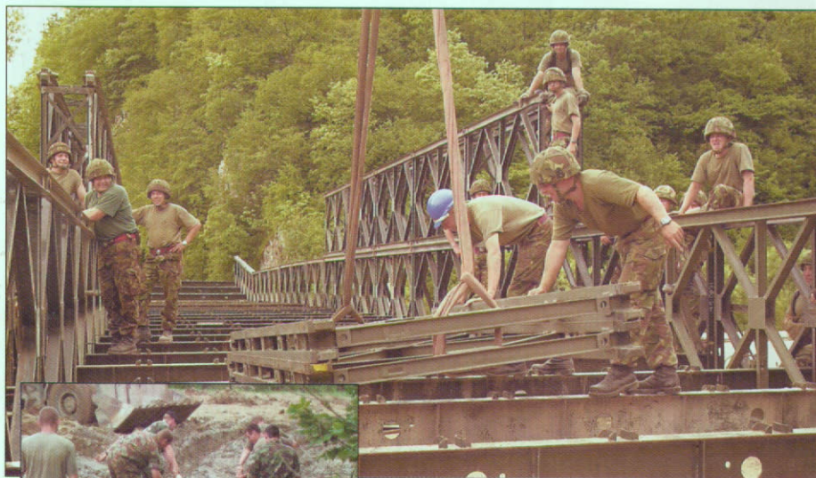
Mind the gap: Sappers, above, constructing the 130ft Bailey bridge at Dabar; and, inset, grateful colleagues assist the project leader, SSgt John Buckley, to celebrate the end of the daunting task
