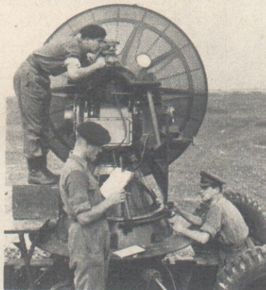
In the guidance area, a Gunner team lays its radar plotter on the Corporal. Computers track the missile in its flight.
