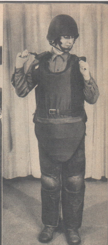
This new body-armor for ground troops to be tried out by Americans in Korea is made of glass fibre, nylon and other plastics. It weighs only five to 15 pounds, according to how much it protects. The helmet is also new and to be tried in Korea. It has an aluminium shell, which can be used as a water container, and a nylon lining.
