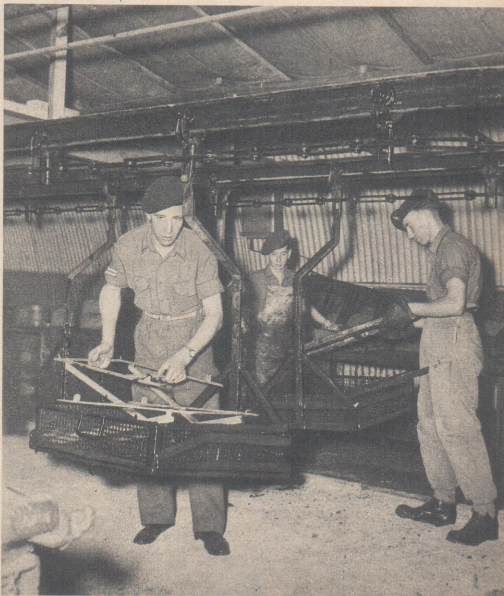
Below: Metal parts take a ride. The conveyor passes them through a tank of "hard preservative" which will last them ten years.
