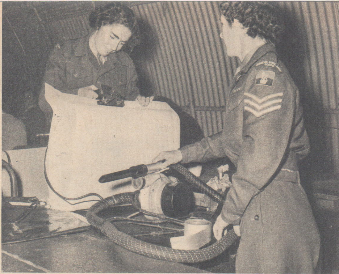
Above: The parcel contains clocks. When the special bag is sealed, except for a small opening, the pump will be used to extract the air. Then sealing will be completed.
