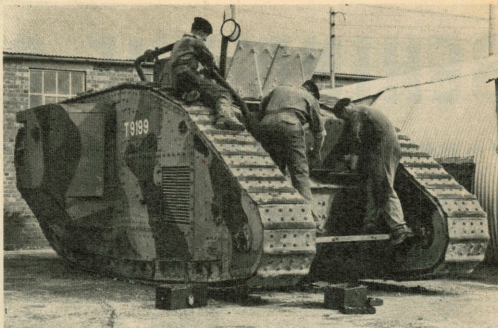
Maintenance work by the School's Light Aid Detachment, REME, on the 1917 Mk V tank, World War One's only remaining "runner." Three men used to turn the engine—now it has a self-starter.
