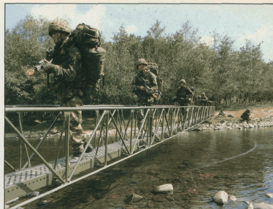
Above – Members of C Company, 7 LI, make full use of the seven-module bridge over a “deep river and gorge” set up for them in half an hour by 7 Pioneer Assault Platoon
