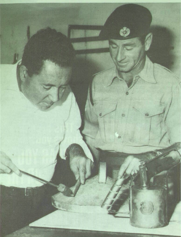
72 Squadron course, St George's Bay: Sgt A Caruana, sheet metal worker and combat engineer, shows Mr J Pizzuto how to solder a container lid.
