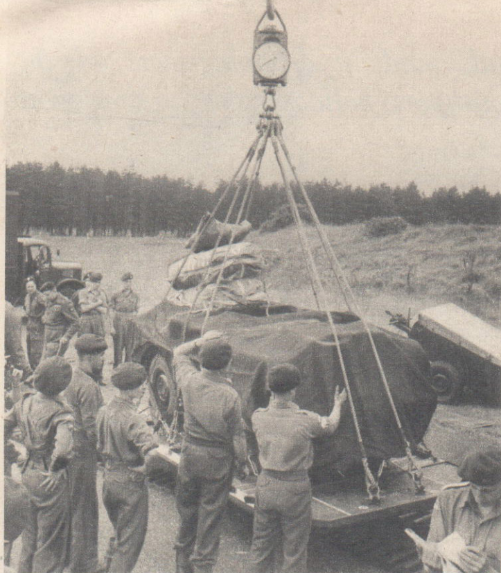
A door is removed from a Flying Boxcar to let a jeep in. Left: The vehicle and its packing are weighed together.
