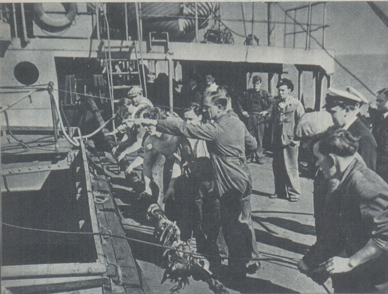
Pluto arrives at the after-hold, preparatory to rewinding.
