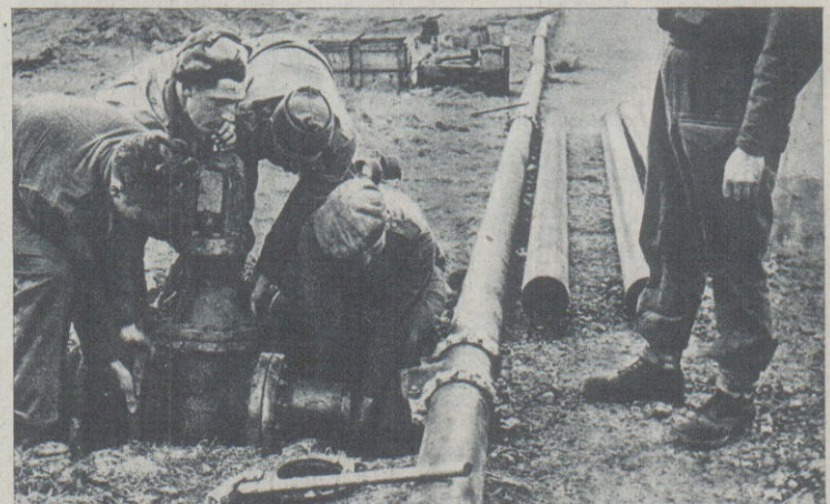
FLASHBACK: October 1944 — British soldiers instal the T-union valve on one of the first sections of Pluto running to Boulogne.
