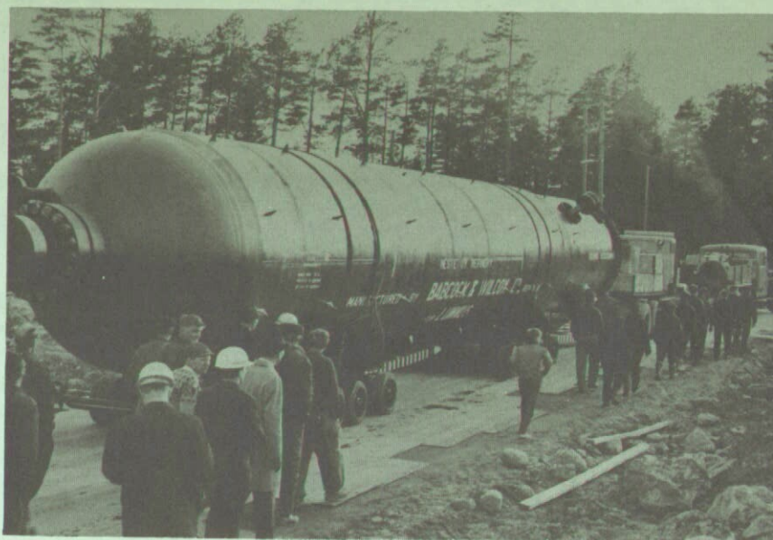
This massive object, pictured being towed away from the coast in Finland, was carried from Britain via the North Sea and the Baltic aboard a Royal Corps of Transport tank landing craft. It is a petroleum reactor pressure vessel built on the Clyde for a refinery near Helsinki. Weighing more than 180 tons, 66 feet long with an internal diameter of eight feet six inches and walls six inches thick, it is the largest and heaviest pressure vessel ever exported from Britain as a complete unit. It is the first time that the Army has ever helped industry by moving a large unit of industrial plant outside British territorial waters. The pressure vessel was loaded and unloaded through the double doors at the bows of the tank landing craft.
