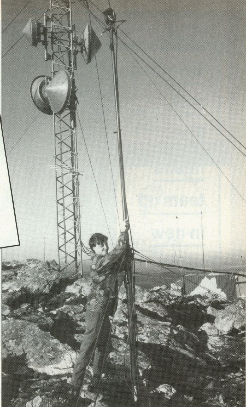
On hill tops where the wind can reach hurricane force, the slightest error in mast siting, or a loose guy rope, can mean a loss of communications. Sig Dave Cooke makes good use of a sunny spell to begin some routine maintenance
