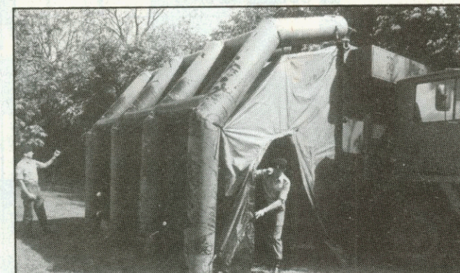
A mobile test laboratory complete with penthouse – SSgt Clive Fenton (left) and Sgt Dave Whalley inflate the struts that support the all-in shelter
