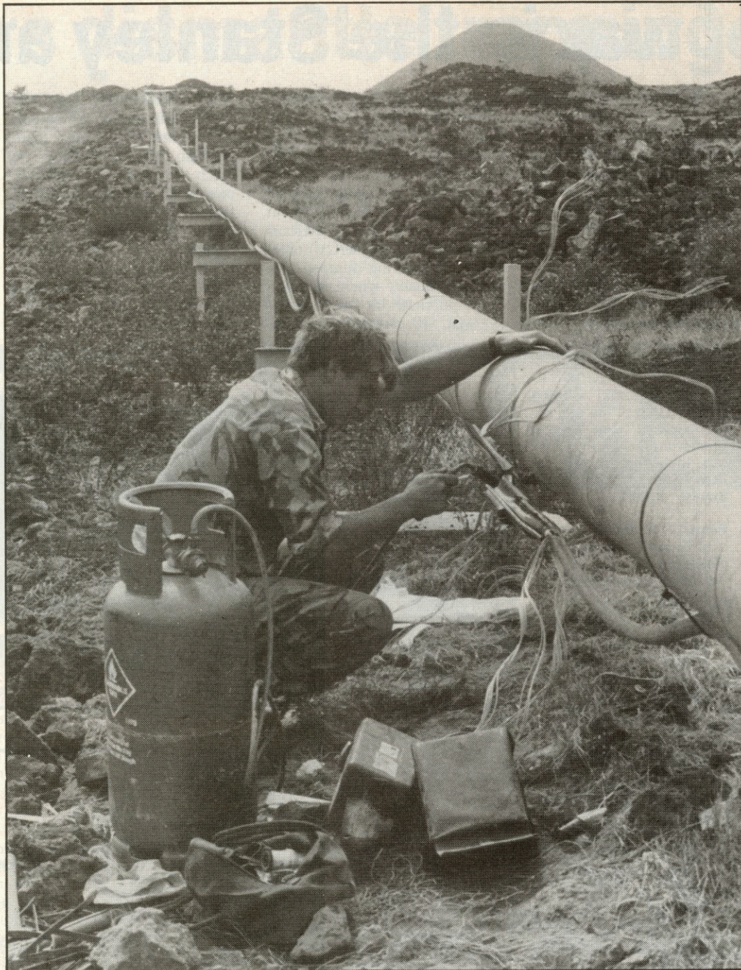
Heat-shrinking a waterproof cable joint hanging beneath the main aviation fuel pipe to the airfields on Ascension Island
