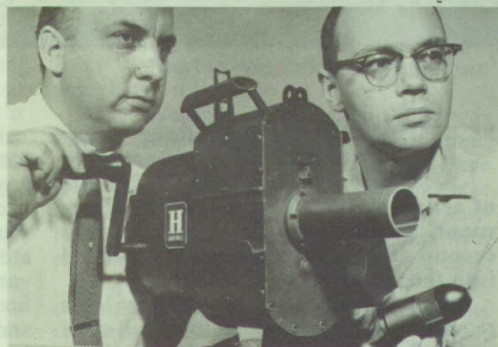
Below: American inventors with a new gun which spits out 40mm grenades at the rate of 250 a minute. It is fired by turning a handle.
