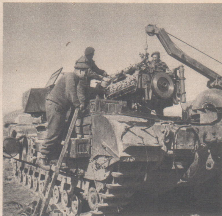
A tank is fitted with a new engine, with the compliments of the Royal Electrical and Mechanical Engineers in Korea.
