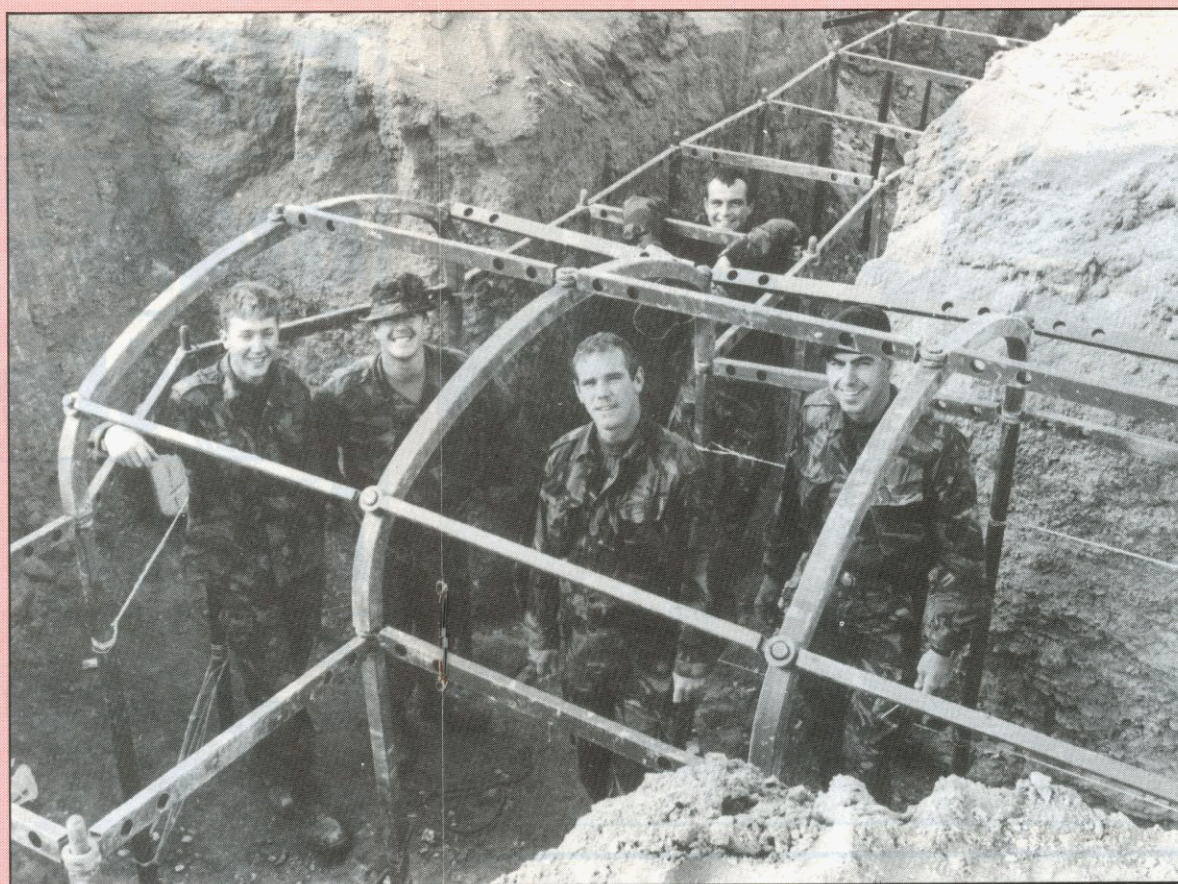
Sappers of 3 Fd Sqn RE from Tidworth construct MEXE shelters
