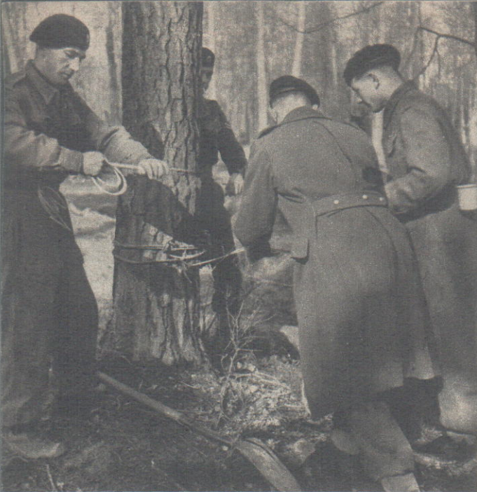
How to demolish a tree in a hurry. A 75 grenade, filled with TNT, is lashed to the trunk (left)... and the result (right) is a mess of firewood. But a lumberjack would shake his head sorrowfully.
