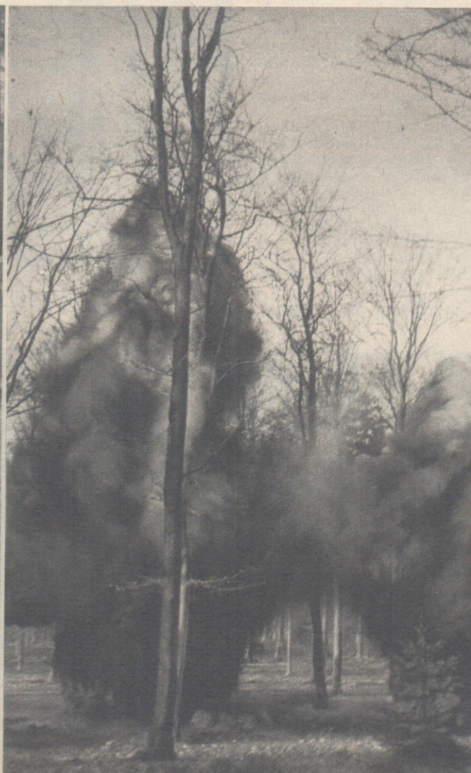
To blow a worth-while crater, first sink your camouflet. For greater effect, craters are blown in pairs (right)...
