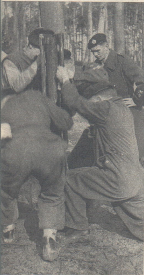
To blow a worth-while crater, first sink your camouflet. For greater effect, craters are blown in pairs (right)...
