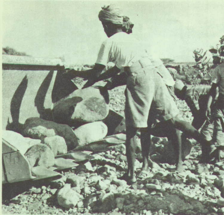
Left: The wadi boulders collected by this coolie gang are crushed and mixed with bitumen as the top surface of the Sapper road.
