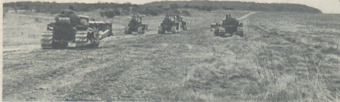
Bulldozer patrol: Sapper drivers set out on the daily job of pushing the landscape back into place. There are miles and miles of anti-tank ditches to fill in along the Southern Downs.
