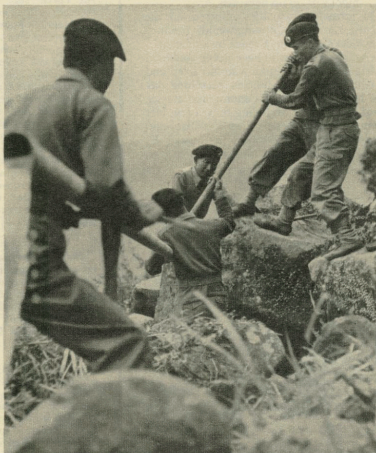
Right: The Hong Kong Chinese add another length of 2½in pipe to the three-mile line which links the dam at Nam She with the villages and Tap Mun isle.
