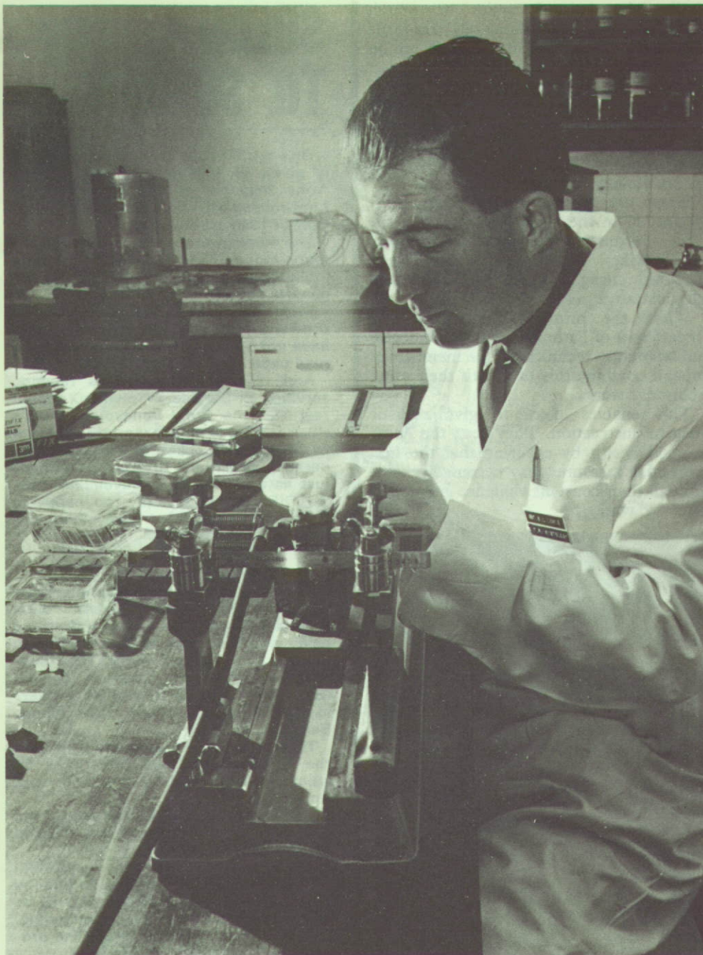
Left: In the Histology Laboratory, Sgt Lewis uses the sledge microtome to cut paper-thin sections from tissue frozen in a jet of carbon dioxide. Above: The end product. Inoculation against 'flu and fevers that attack the soldier and against which he would be defenceless.
