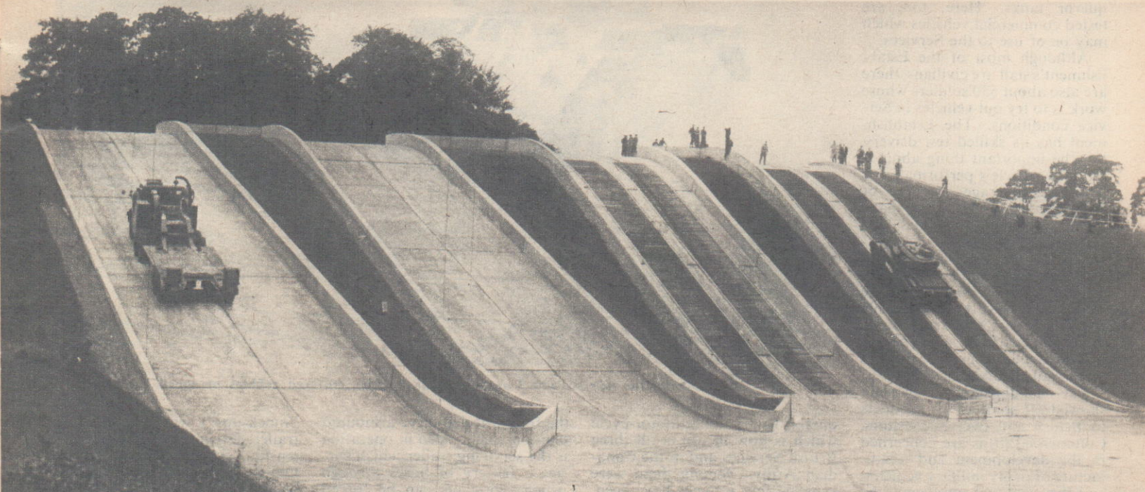
The imposing array of test slopes: Gradients range from one in four to one in 1.73.
