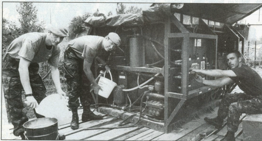
This NBC 6 water purification unit is providing washing and drinking water for the British base at Vitez. Checking its chlorination levels are Sprs Harry Chapman, Dutch Holland and Brian Girdwood
