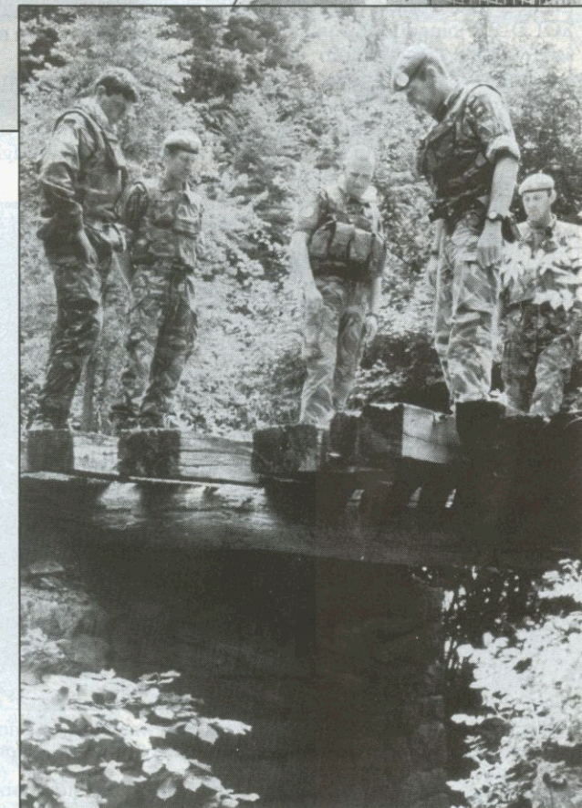
Will this rickety wooden bridge bear the 30-ton weight of a Warrior infantry fighting vehicle and its ten-man crew? The sappers must decide
