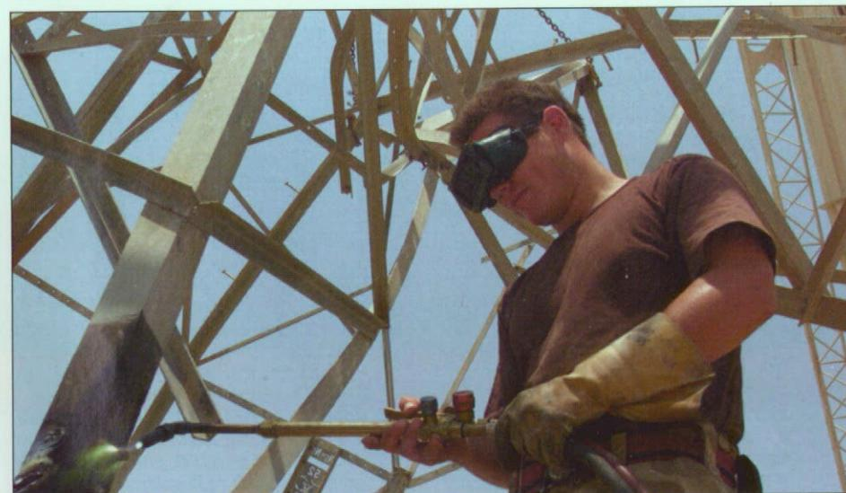
Spr Glen Parker, a welder serving with 15 Field Support Squadron, part of 38 Engineer Regiment, cuts bolts off a badly twisted section of a power pylon damaged by copper thieves. Crime like this is making it difficult for coalition forces to provide local communities with electricity
