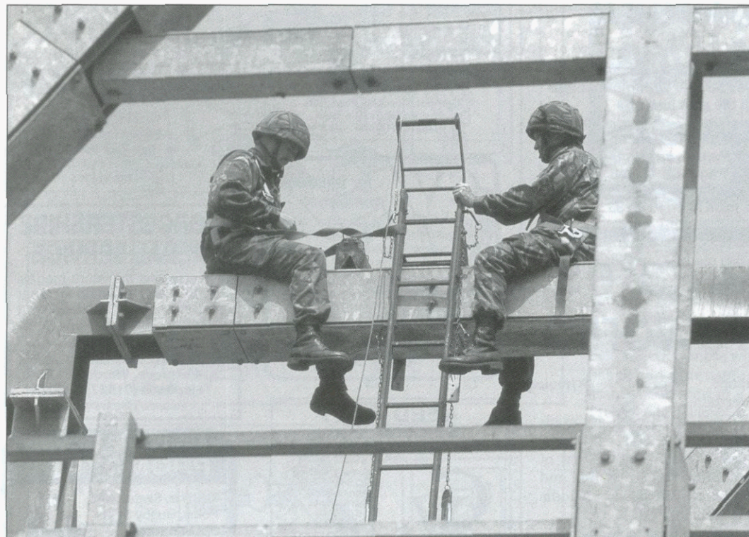
Soldiers of 100 Fd Sqn, R Mon RE (M), place demolition charges on a heavy girder overbridge this year
