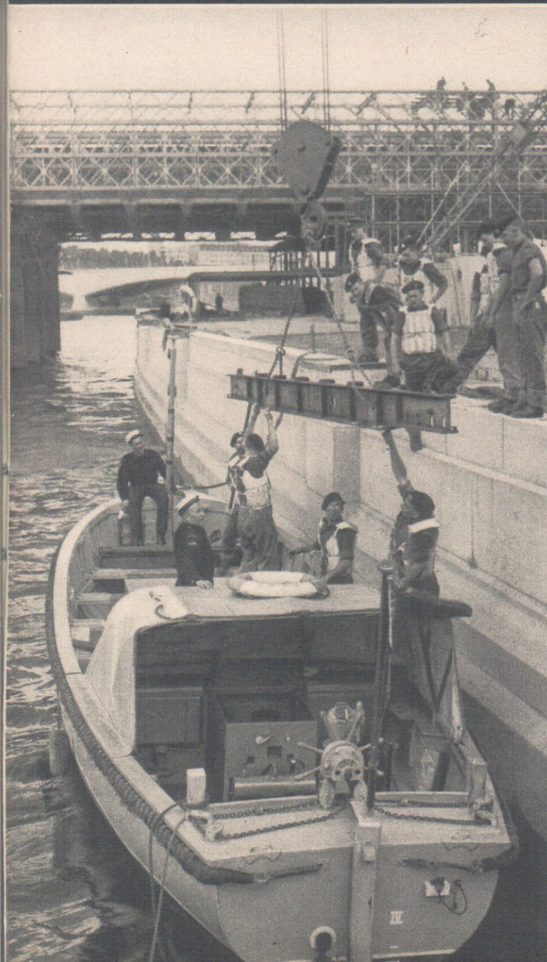
Lifting the first section ready for launching the first span of the bridge. Below: a girder goes by RASC launch to the men working on the north end of the bridge.
