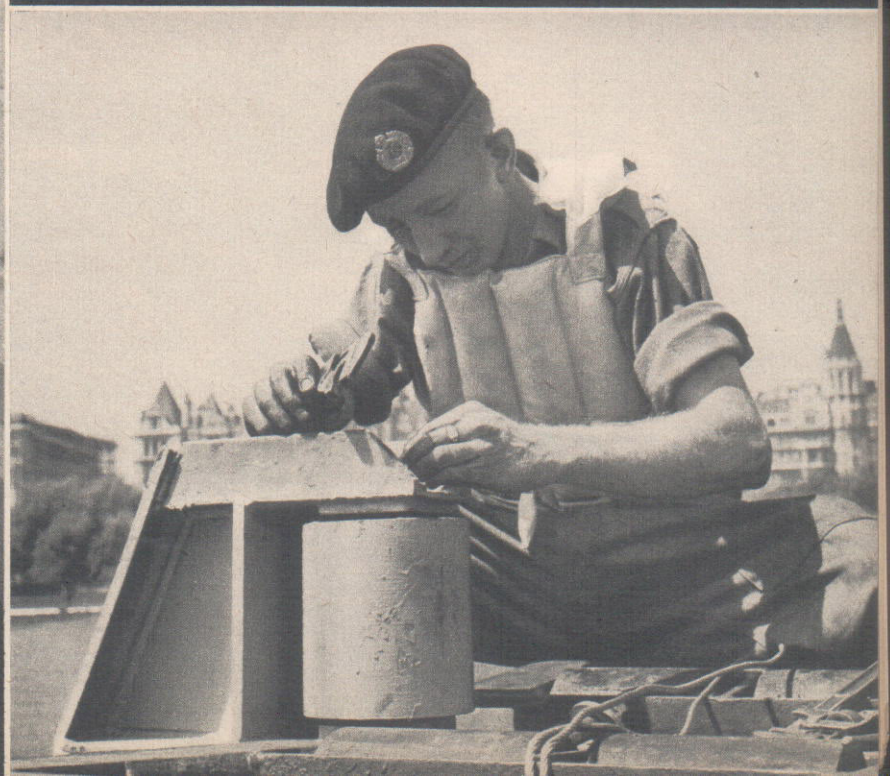
The bridge is almost across, and transoms are being fixed into place. Below: Sapper Kenneth Excell wore a life jacket when he assembled roller bearings on top of a pier for support of the bridge.
