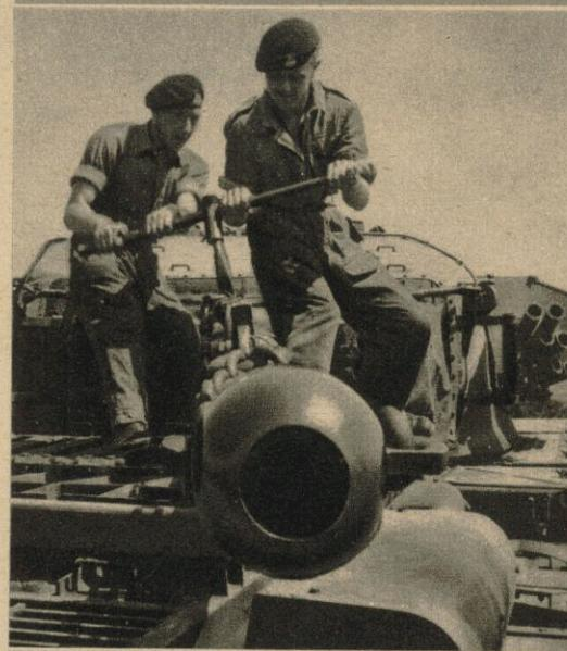
With the aid of a chain, lever and ratchet the gun barrel is pulled back, then a quick-release device lets it run out: Troopers R. Abberley and J. Neave on the job.
