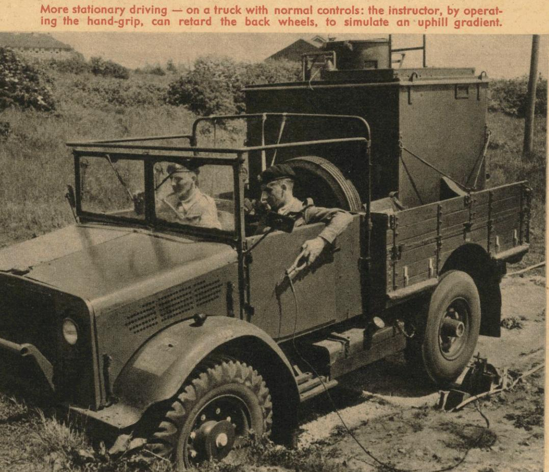
More stationary driving — on a truck with normal controls: the instructor, by operating the hand-grip, can retard the back wheels, to simulate an uphill gradient.
