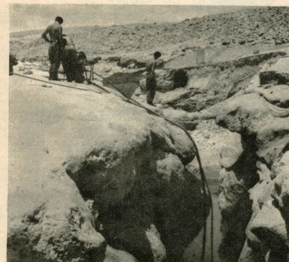
Left: The Sappers had to find their own water—in this instance from an almost dried up wadi. The water was pumped up to purifiers and within a few hours it was fit for drinking.
