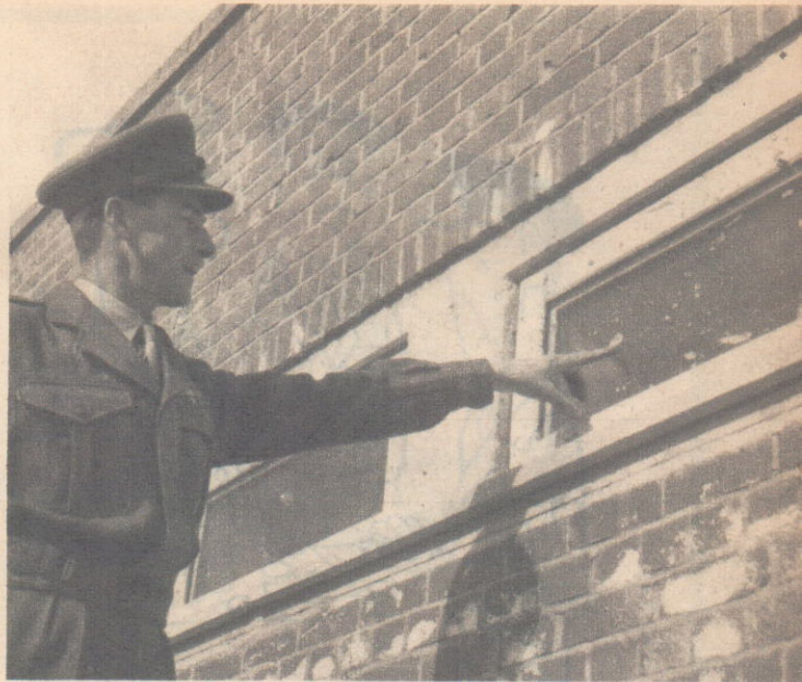
To test delay fuzes the fuze range is marked off in scores of yards. Right: Shatter-proof glass peepholes are fitted in all the firing shelters. Pock-marks show why.
