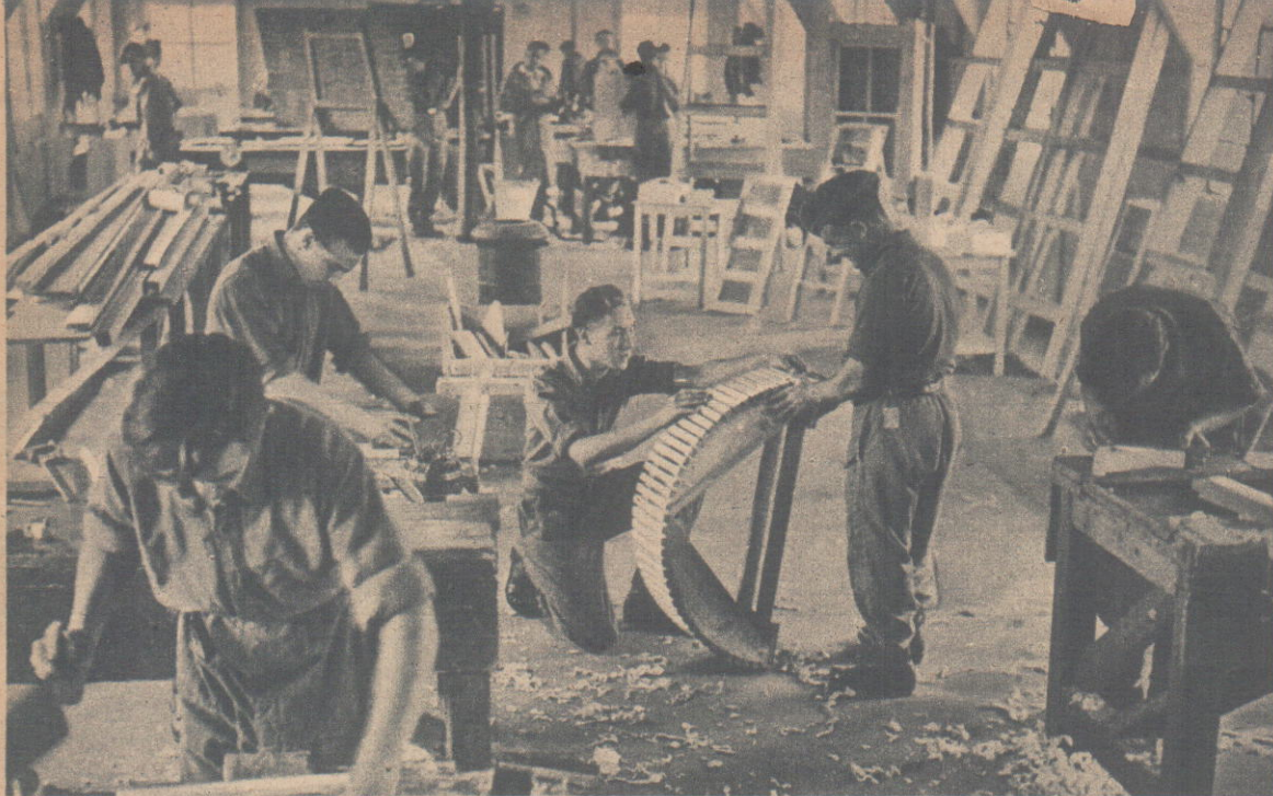
The carpenters' shop. The arch-form will be used by student bricklayers building arches.
