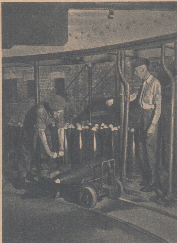
Above: ammunition in a chamber below a 9.2 is wheeled on a circular "railway" to the hoist, which traverses with the gun. Below: The 9.2's, like this one, in the Dover area have a range of more than 30,000 yards and blasted at German shipping during the war.
