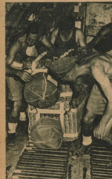
Panniers roll to the open door of the plane on a roller conveyor. This method, with slick drill, gets eight panniers away in as many seconds.
