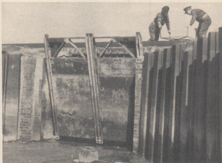
Bailey Bridge panels keep out the Medway's flood waters.
