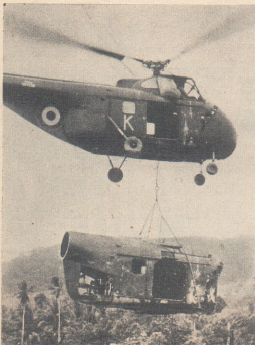
Helicopter saves helicopter. The first machine made a forced landing in an inaccessible paddy-field, was dismantled and retrieved by a sister aircraft.
