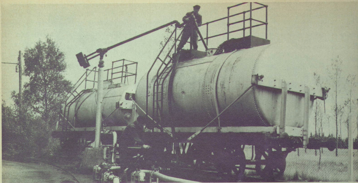
Loading a rail tank car with diesel fuel at the centre's practice training pipeline.
