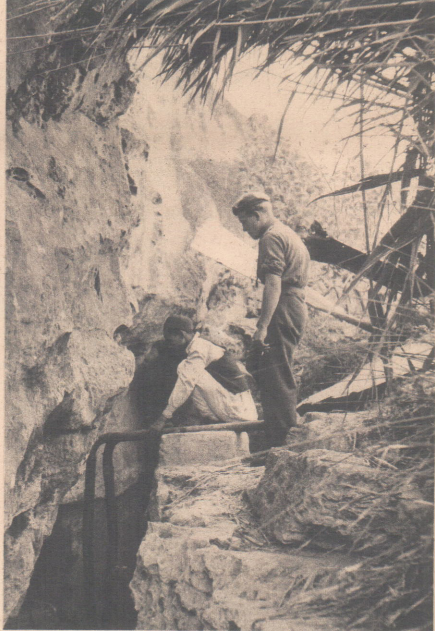
Private Frank Rowley of Lambeth has started the pump at the oasis. With him is the khaffir who guards the spot night and day. Left: Examining the pipe line which brings the water from the oasis to the laundry: Corporal George Naisby.
