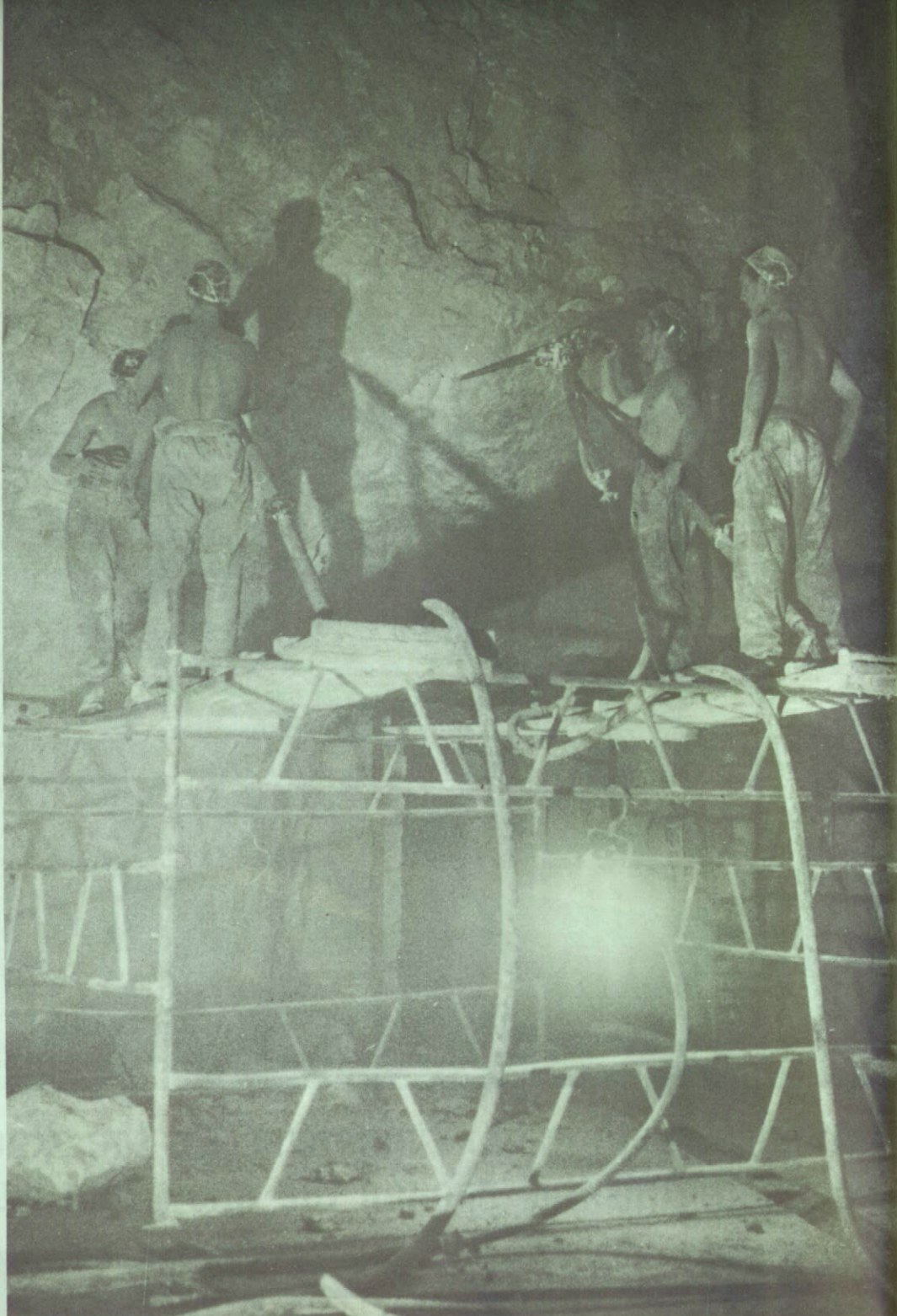
Above: In 1948 a SOLDIER cameraman took this picture of "Moles" at work in the Rock. Two drillers are making a hole for a charge. In civilian life one had been a miner and other other a steel worker.
