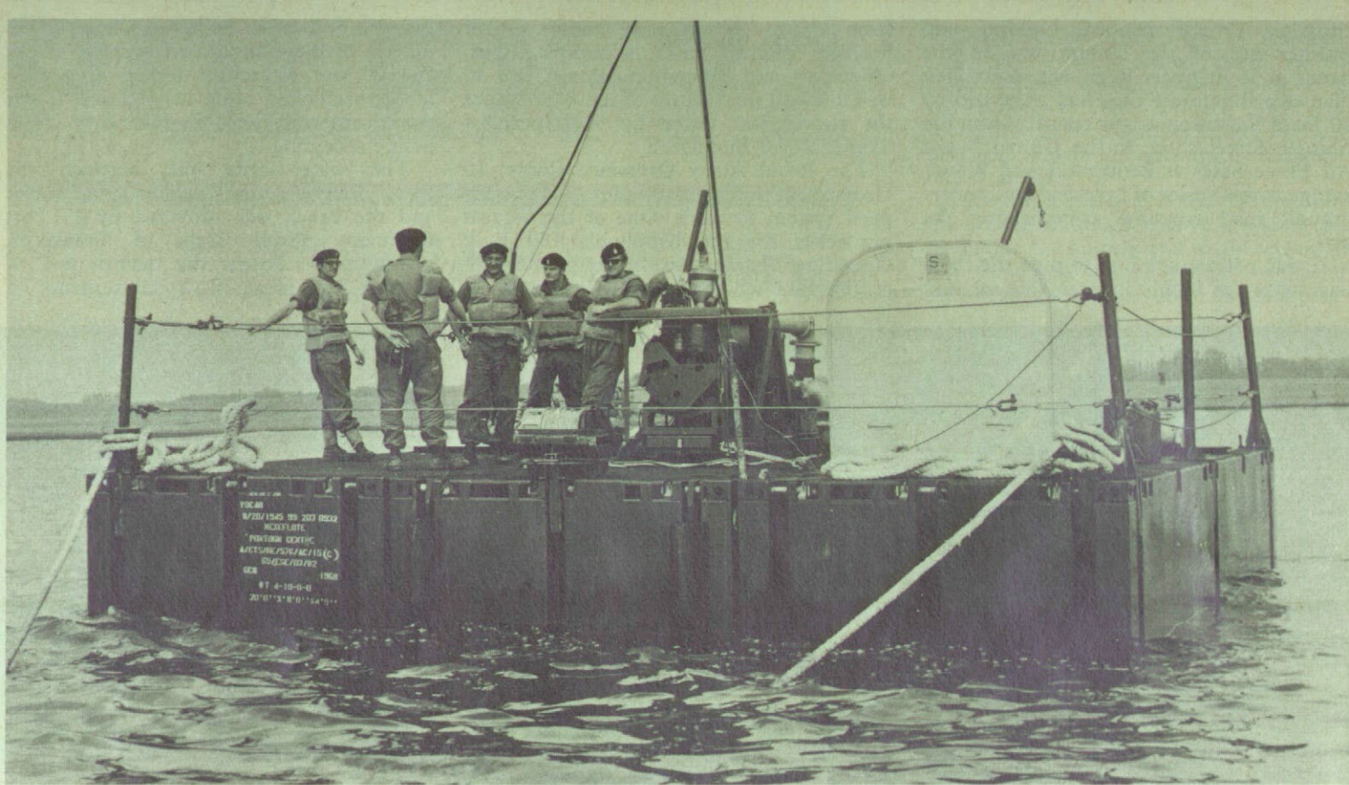
Above: The Mexeflote pontoon carrying the flexible pipe which takes fuel to the beach.
