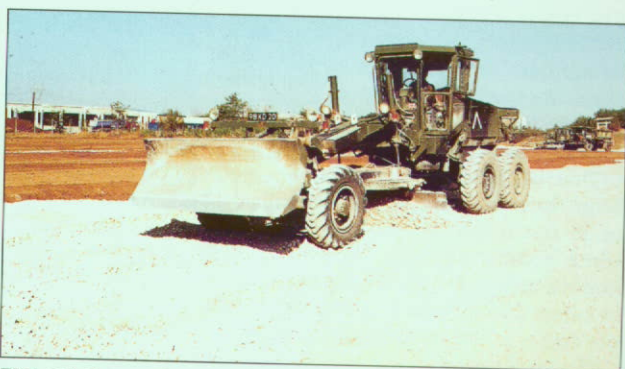
Flat-out: A squadron grader spreads crushed stone at the temporary field accommodation site on the outskirts of Pristina
