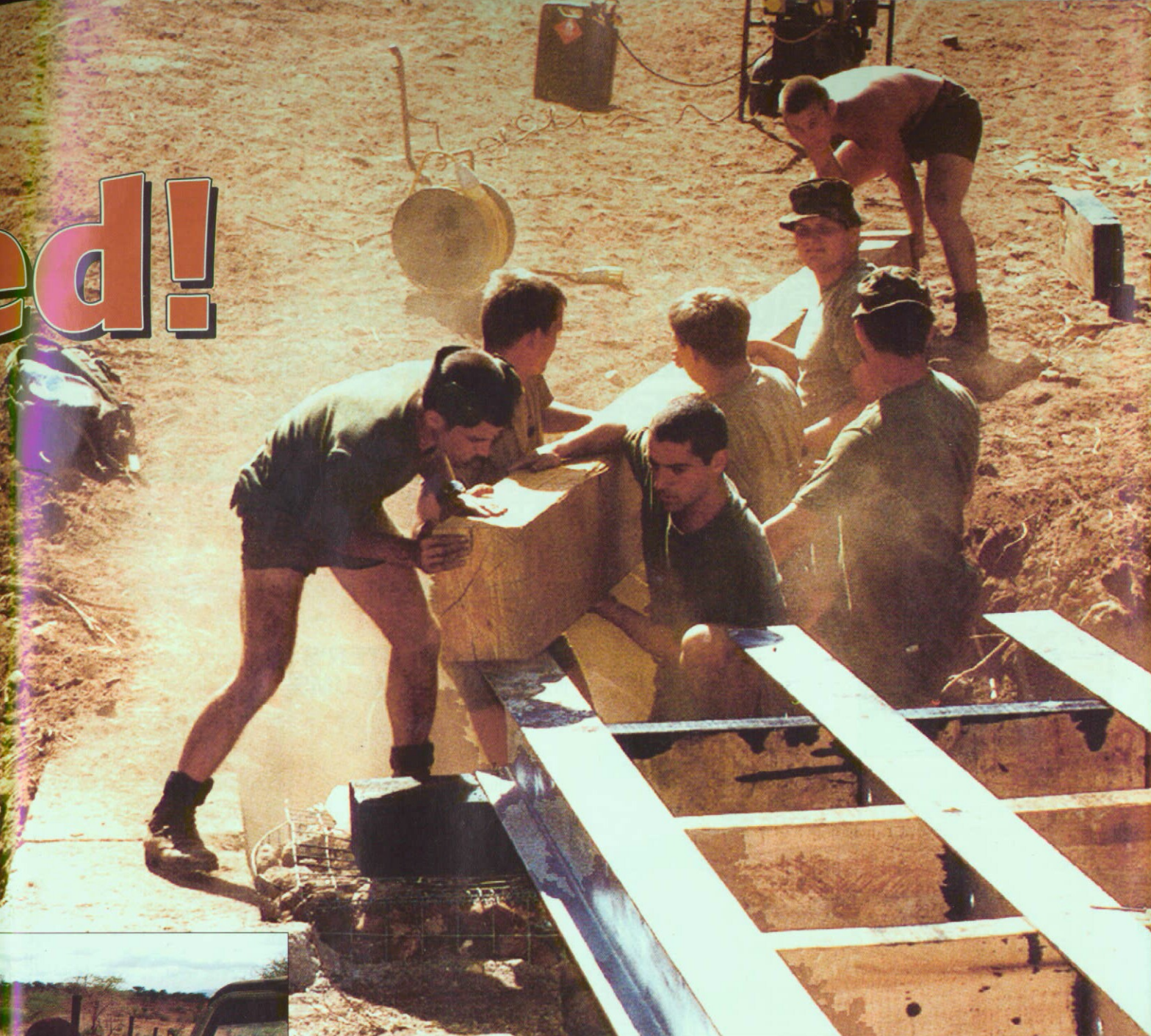
Hot work: Sappers, right, manhandle an 18ft solid wooden beam into position on one of the new bridges
