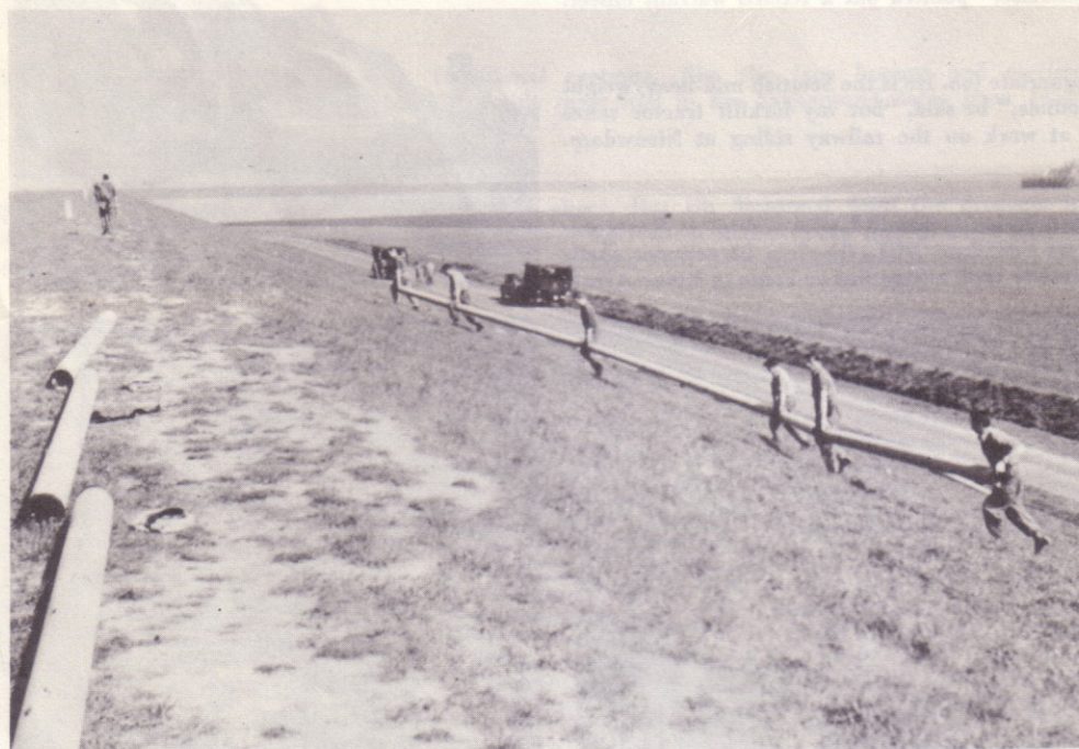
Below: Laying the pipeline. It was 6½ miles long and took less than a week. Through it were piped 400 tons of diesel fuel which had to be shipped back to Britain—normally it would have been aviation fuel for the RAF. TAVR men who built the pipeline included qualified civil engineers.
