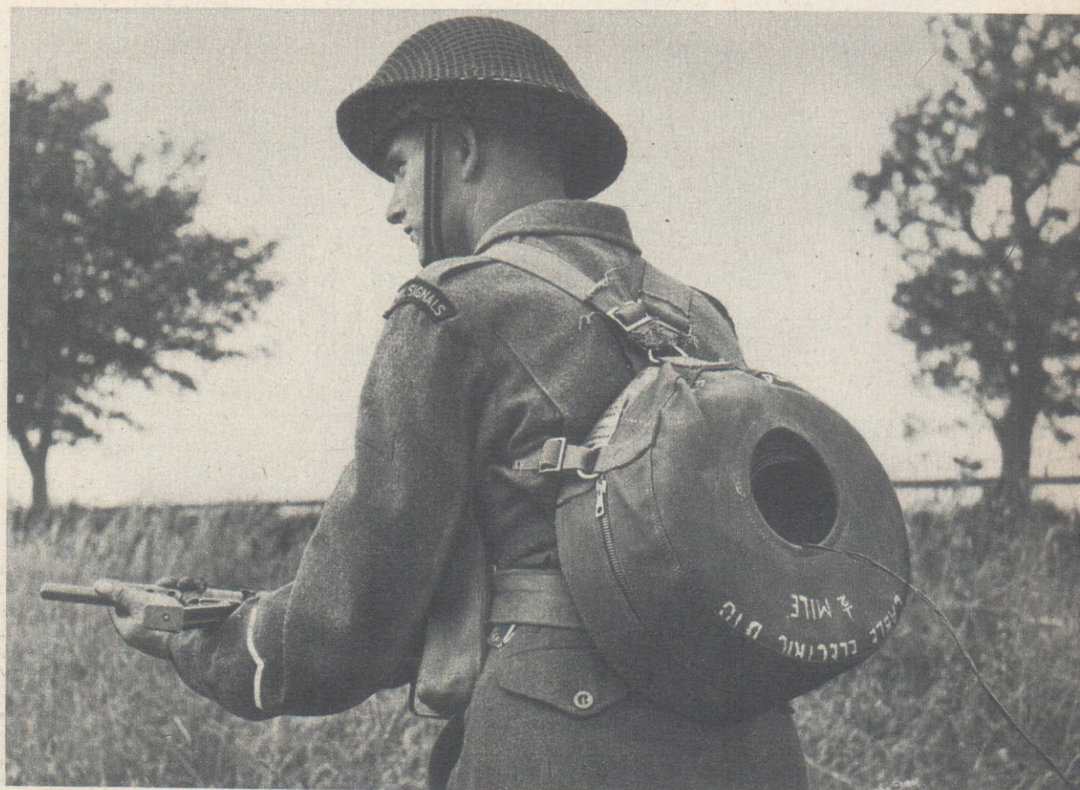
Below: The cable unwinds itself, like a ball of string, as the lineman walks along, leaving his hands—and eyes—free.
