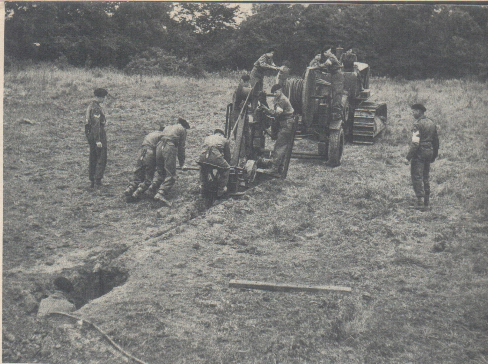
The cable-laying plough in action. Note the narrow furrow which soon becomes almost invisible from the air.
