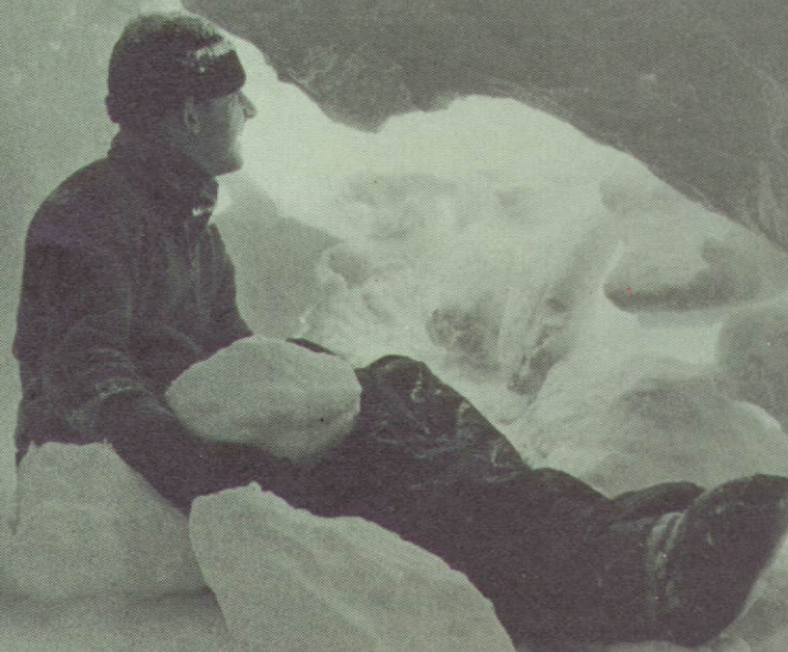
First you dig your hole in the snow; then you plug up the opening (remember first to dig a separate entrance tunnel). A bombardier of the Force Artillery's potential Arctic instructors course working on the inside.
