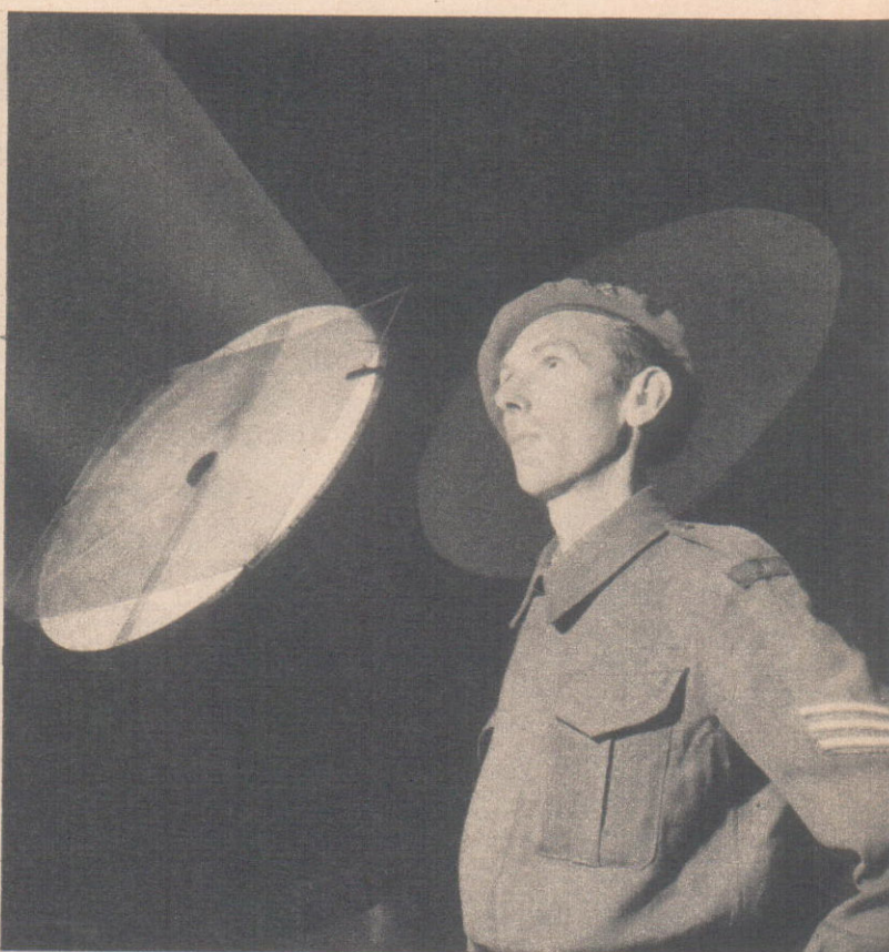
Serjeant J. Ogilvie, detachment commander, observes the beam. The halo behind his head is the radar aerial, mounted beside the searchlight, which has a coloured screen to avoid dazzling the pilot of the target aircraft.
