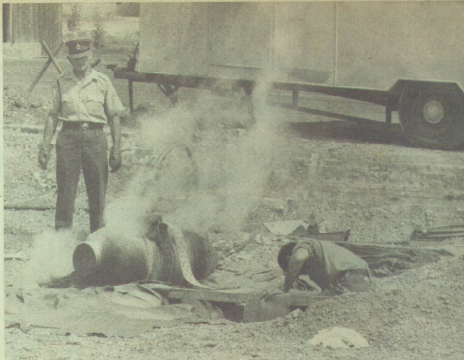
Army bomb experts Captain John Dickson (left) and Corporal Eric Meagham steamed explosive from a 1200lb German bomb found in a council yard near Bexleyheath Broadway. The
