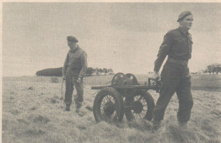
Across the bleak downs of Larkhill ranges, men of the Range Detachment lay telephone cables for practising units.
