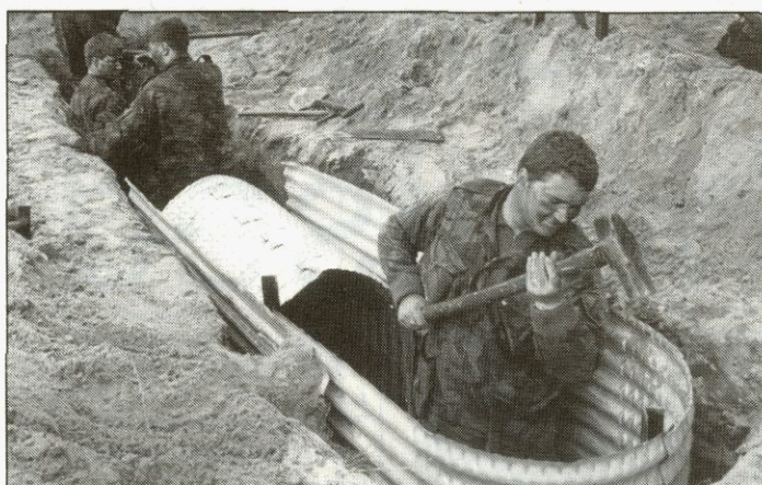
Cpl George MacFarlane (right) knocks up a defensive position using a flexible trench support system
