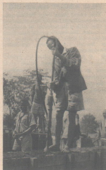
Pounding the earth between the shutters to make a hard-soil wall.
