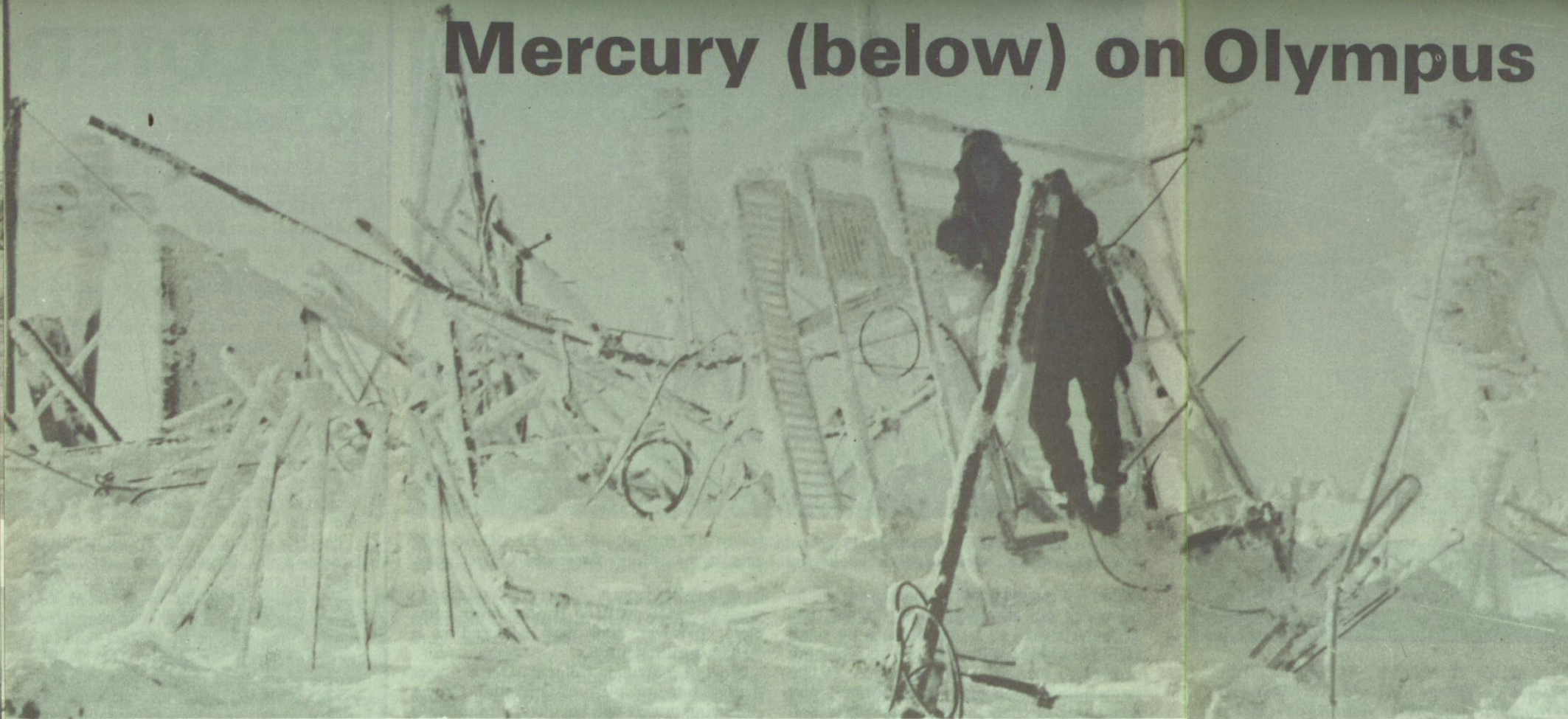
A Mount Olympus blizzard reduced a 60-foot signal tower to ice-coated wreckage.
