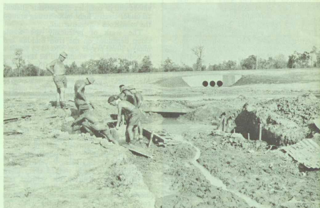
Above: Stone and bitumen are fed into Starmix 8 to produce about 100 tons of asphalt per shift. Below: Working on a culvert. Drainage was a major problem of the runway (background).
