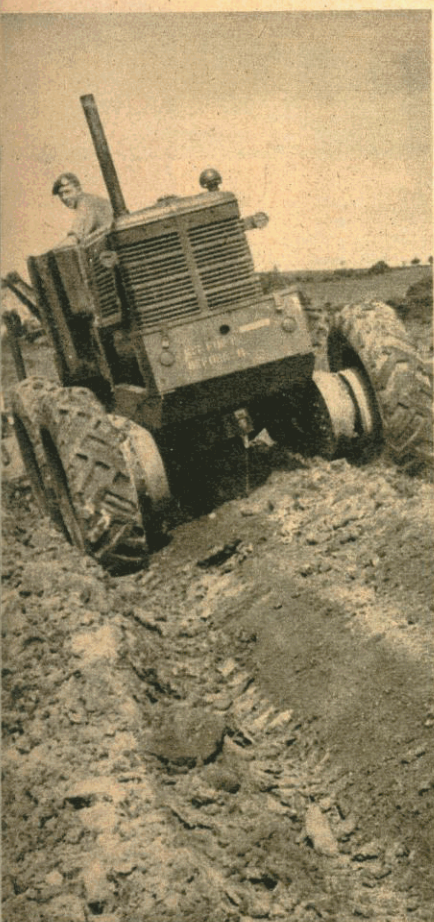
This grader is cutting a drainage ditch at the side of the highway.
