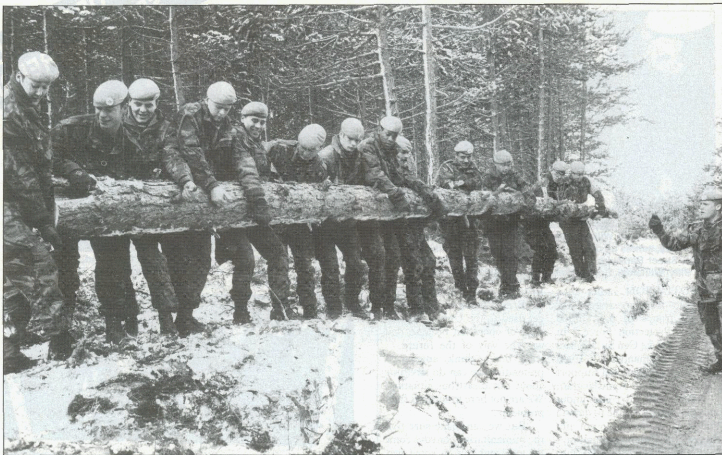
Sappers from 35 Engr Regt use local timber to make repairs to main supply route Triangle above Tomislavgrad
