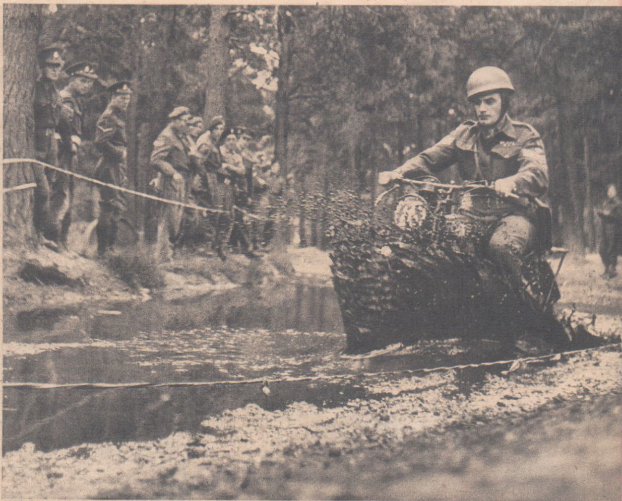
Above: The right way... This REME Staff-Sjt. first tested the water-splash on foot, then drove carefully over the firm patches. Below: The wrong way... He didn't paddle through before riding into the water. He will paddle out with a drowned engine.
