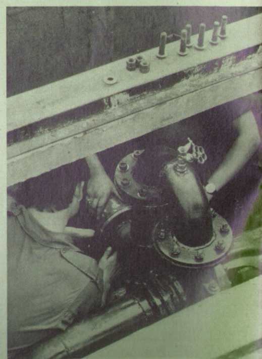
The tank washdown filter system is put in place.
